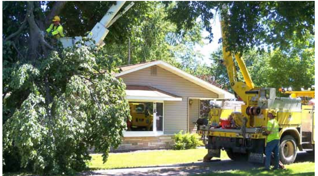
Line crews worked around the clock from July 1-3 to restore power. A number of downed trees slowed their progress.
