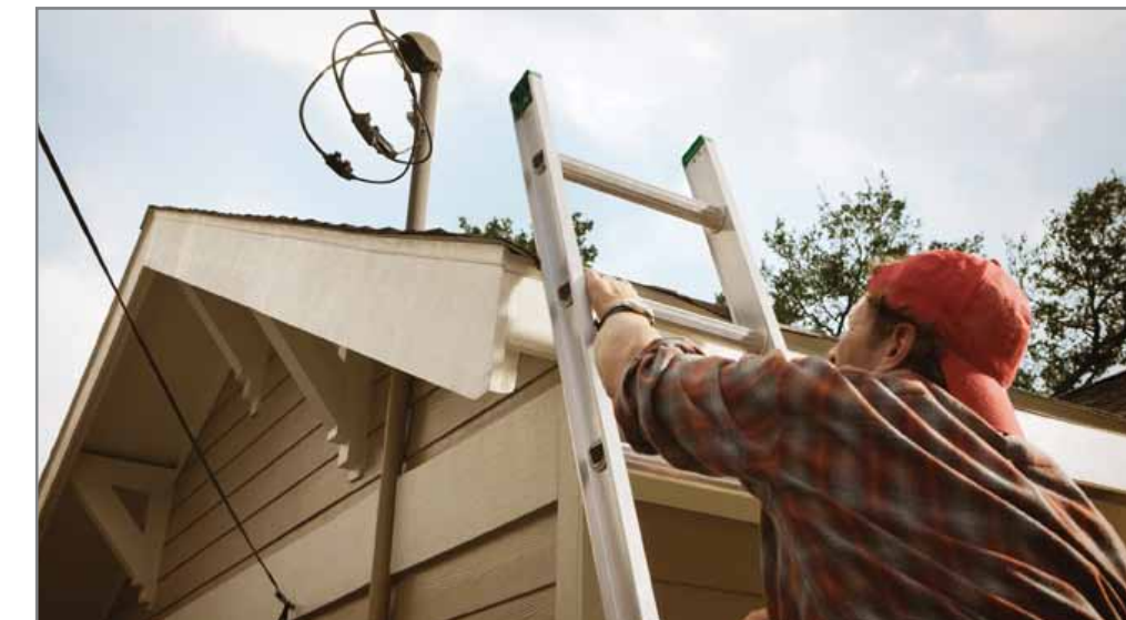
The general public should always stay clear of dangerous overhead power lines, and take caution when using tools such as ladders and scaffolding around them.
